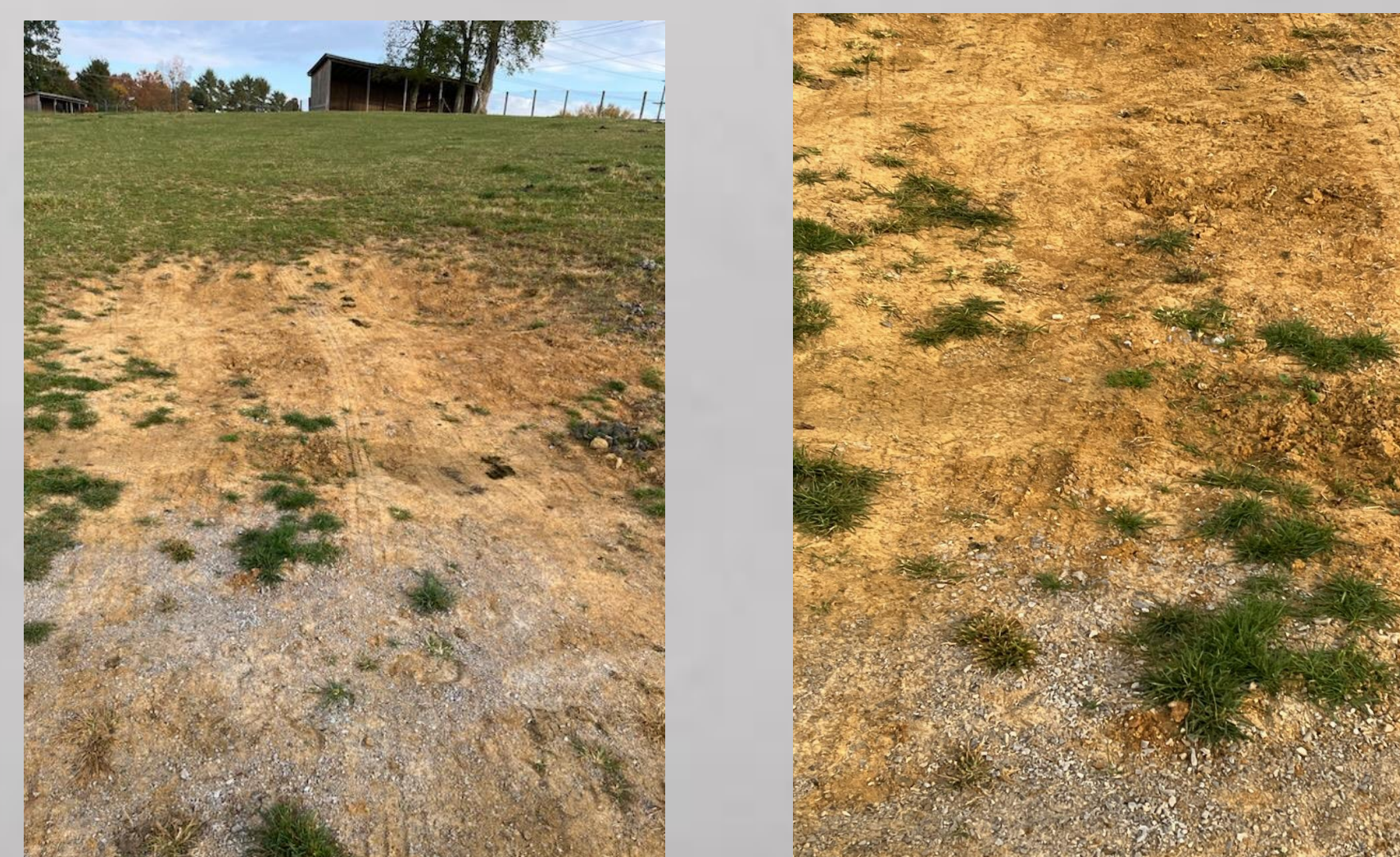
These two images show the drain 5 weeks after installation
