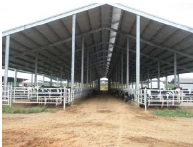
Vanderhyde Dairy – Chatham, VA
